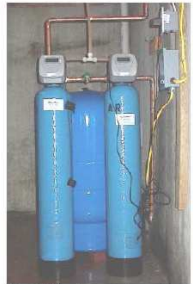
Use of AD33 media in typical point-of-entry system installation. Picture courtesy of Aquamech, Inc.
